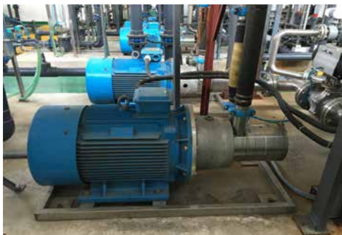
RO plant with two trains - each using two APP 30 pumps
