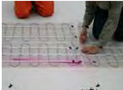
DSVF-90 (DEVIheat™ 90S) mat is laid out.
