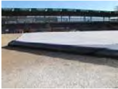
Drainage mat, directly on soil.
