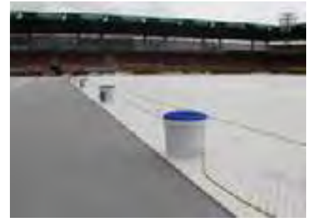
Shock pad, laying out
