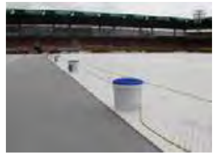
Shock pad, laying out
