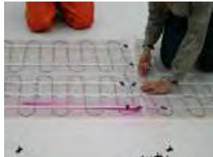
DSVF-90 (DEVIheat™ 90S) mat is laid out.
