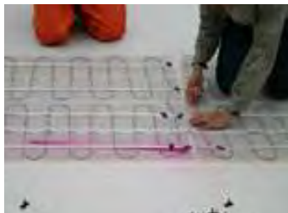
DSVF-90 (DEVIheat™ 90S) mat is laid out.
