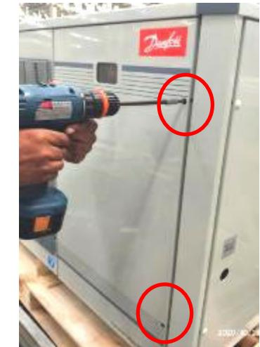
Close the side panel & tighten 2nos of screws
