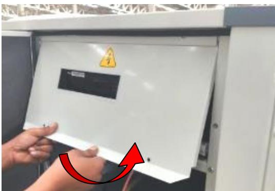
Reassemble Electric Box cover & tighten 2nos of screws
