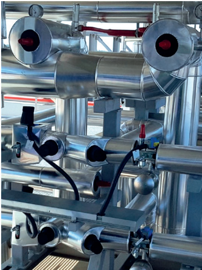
Fig. 2. Evaporator valve stations under thermal insulation.
