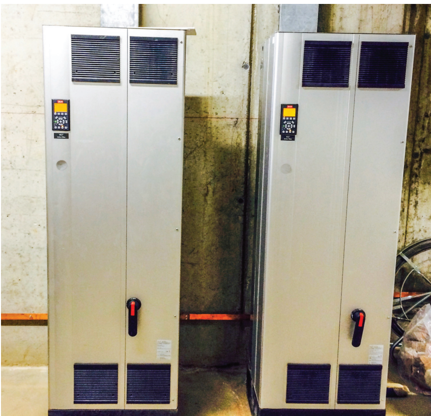
Two VLT® Advanced Active Filter AAF 006 400 A
