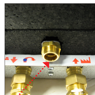
Circulation pipe connection
