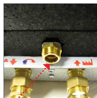
Circulation pipe connection
