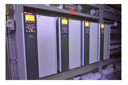
The VLT® HVAC Drive guarantees energy-efficient operation of fans, centrifugal pumps and compressors, for example, and offers perfect EMC properties as a result of the integrated chokes and high-quality EMC filters.
