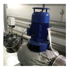
The drive reduces the speed of the process water distribution pump, which in turn reduces heat loss. In addition the insulation reduces heat loss even further, resulting in a double energy saving.
