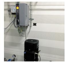
VLT® AQUA Drive controls each pump for central heating water distribution, reducing energy consumption by up to 40% compared to direct-on-line operation. The process water pumps at a rate of 250-350 m<sup>3</sup>/h
