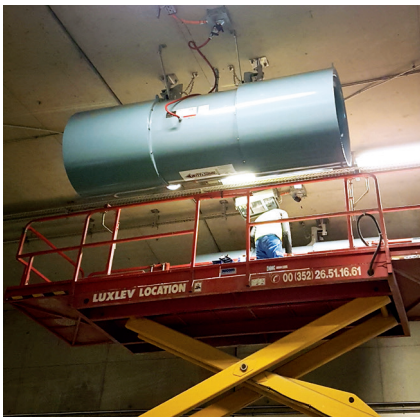
Working on a ventilation unit.
