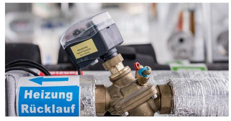
AB-QM balancing and regulating valve allows precise control of the water flow and reduces energy consumption.
