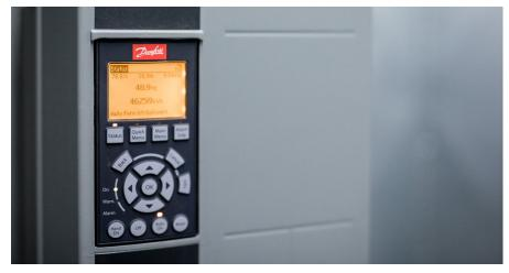
With frequency converters, the fans of the clinics' air-handling system can be operated up to 40 per cent more efficiently.
