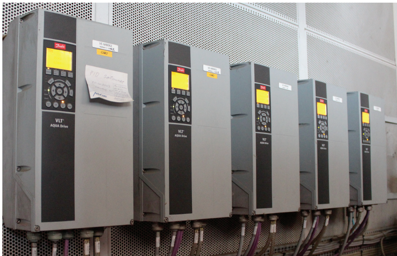
Biogas power generation: VLT® AQUA Drives control cooling fans and booster plant.
