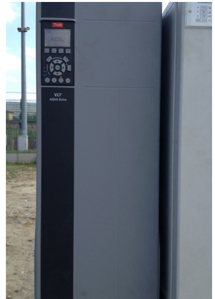
VLT® AQUA Drive FC 202 IP66 frequency converter installed outdoors, adjacent to the water collection tank
