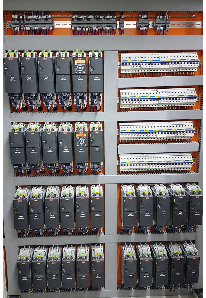
In total, the biscuit factory boasts 100 installed VLT® Midi Drives, controlling equipment as varied as fans, conveyors and mixers.
