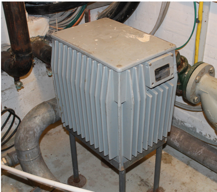
This VLT® 5 drive model in aluminium housing was introduced in 1973. At the Municipality of Tønder in Denmark it has ensured reliable, low-energy ventilation for more than 40 years.
