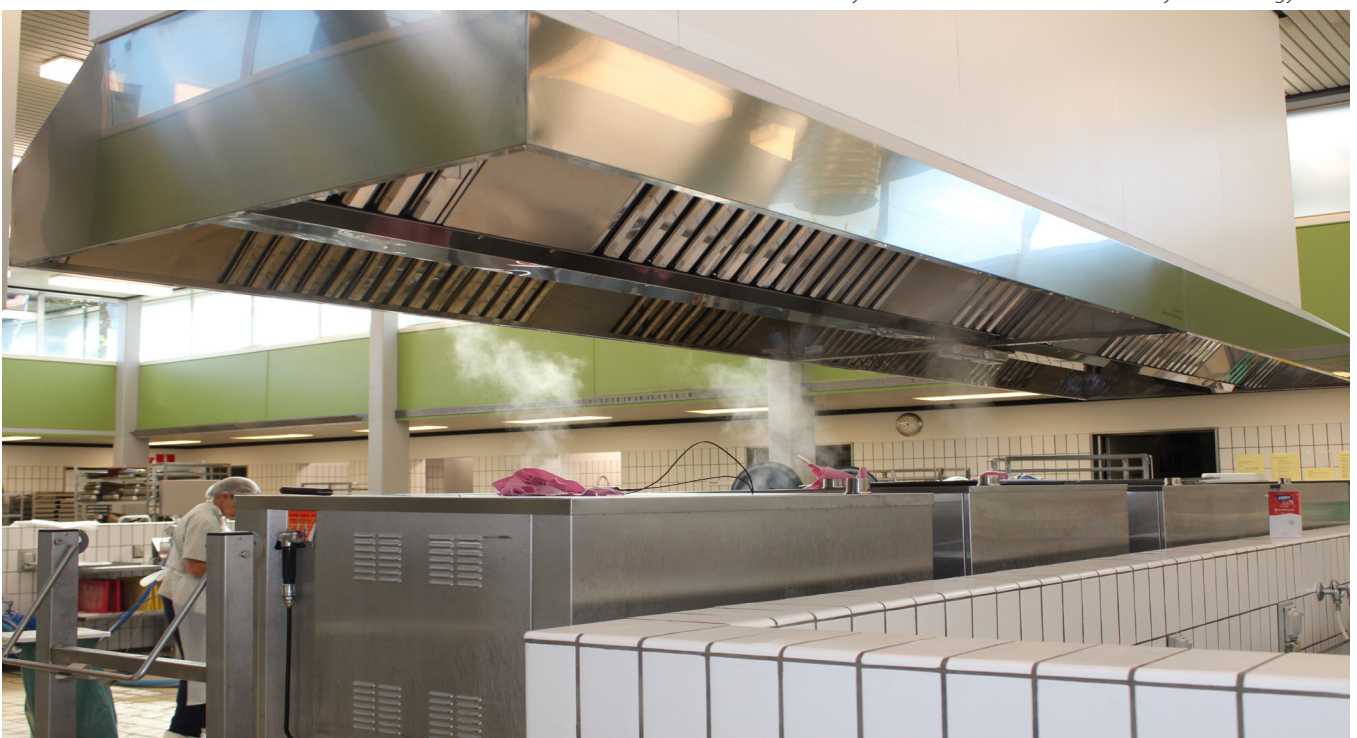
The new ventilation system includes a renovation of the ventilation room for the industrial kitchen, as well as a new ventilation system for the basement and nearby dermatology clinic
