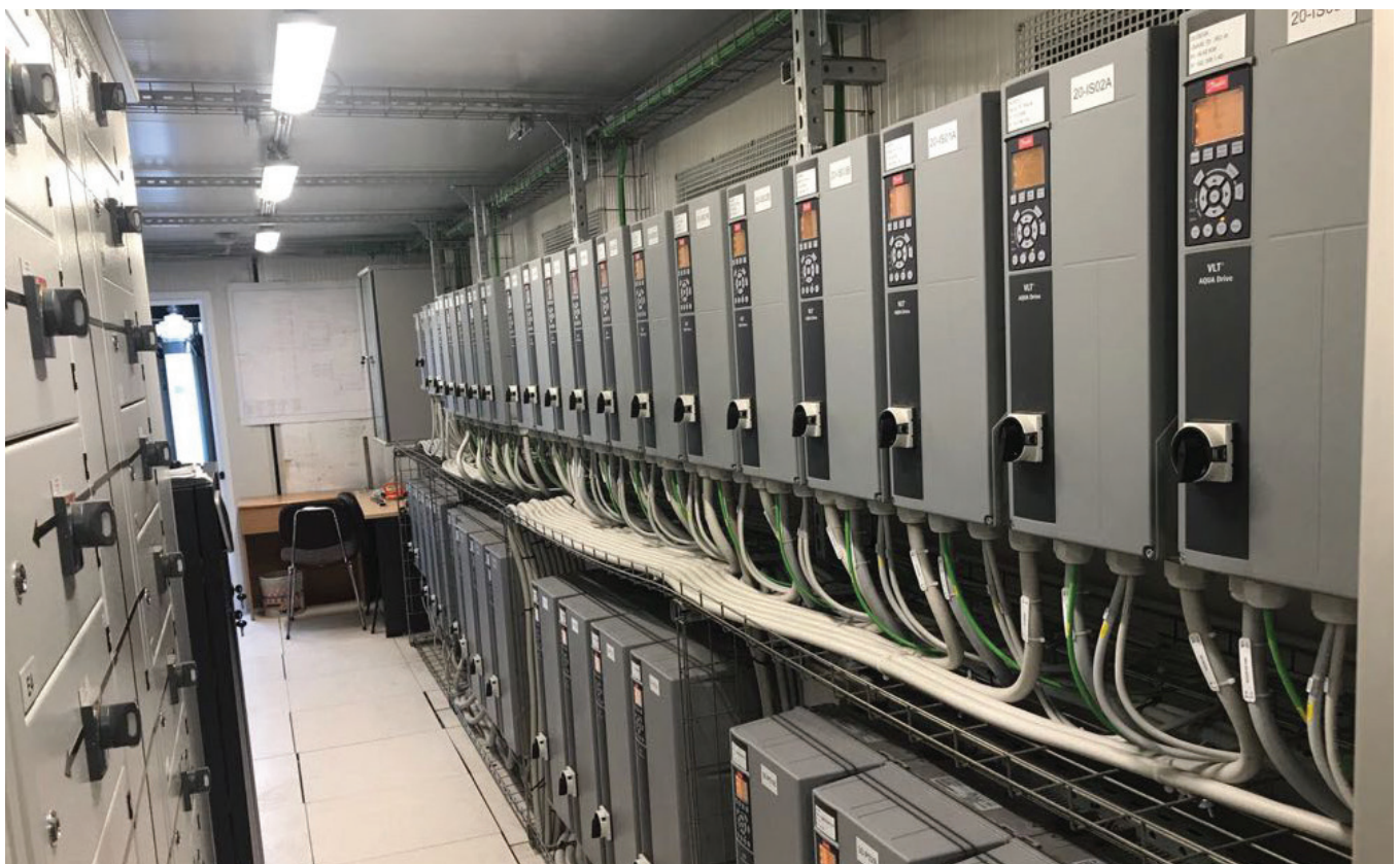
Acciona has optimized the overall efficiency of the plant and the space occupied inside the containers, thanks to the unique compactness of VLT(R) AQUA Drive.
