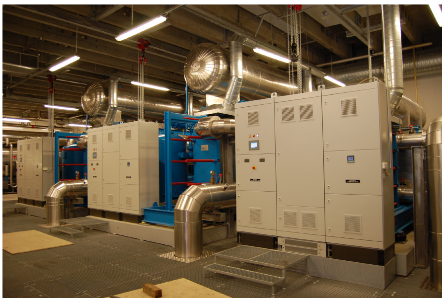
The refrigeration system comprises two 3.5MW screw compressors and one 1.3MW reciprocating compressor.
