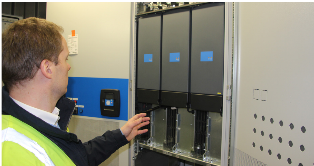
Sverre Knapstad, Frekvensomformer.no demonstrates the VACON® NXP modules installed inside the container
