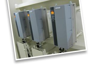
"By using Danfoss VLT® drives, pumps operate consistently at their optimum level for cooling, to save energy. The same principle applies when using these drives in air-conditioning systems,"
