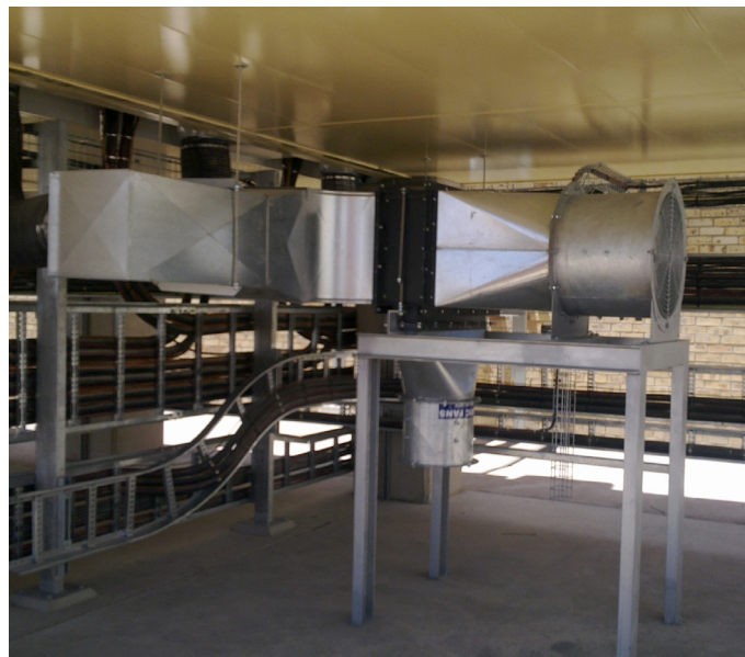
Maintenance-free spin filter system removes dust from air before it enters the heat sink channel of the frequency converter.
