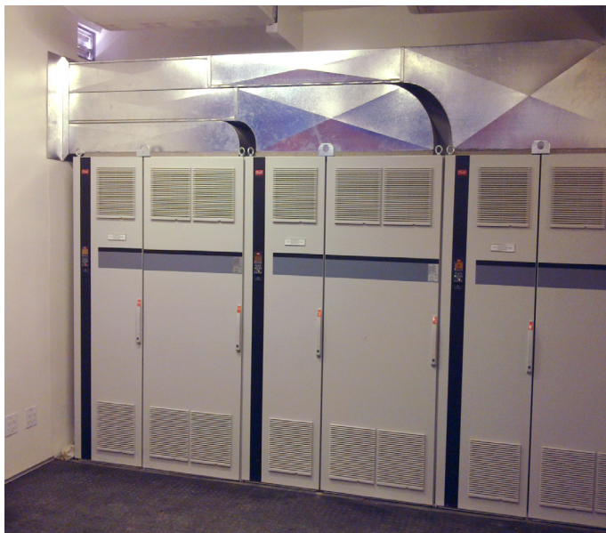
These VLT® AutomationDrive frequency converters with back channel cooling control motors in the mine dewatering system. They are installed in the MCC substation.
