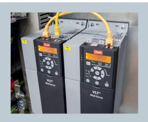
Tresch Automation chose the Danfoss VLT® Midi Drive FC 280 to control the speed of rotation which is defined by the system. The winemaker can then adjust the speed up or down by a few percent using a keypad.
