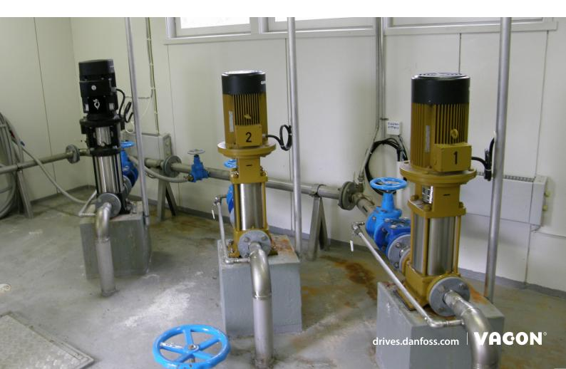
VACON® 100 FLOW drive, and a separate contactor unit is no longer needed. At the Osvald waste water pumping station, direct on-line starting was previously used to start the pumps. This caused a pressure spike in the pipes and mechanical stress on the equipment. After modernization, the VACON® 100 FLOW units accelerate the pump motors quickly but smoothly to their running speed, avoiding extra mechanical stress on the parts.
