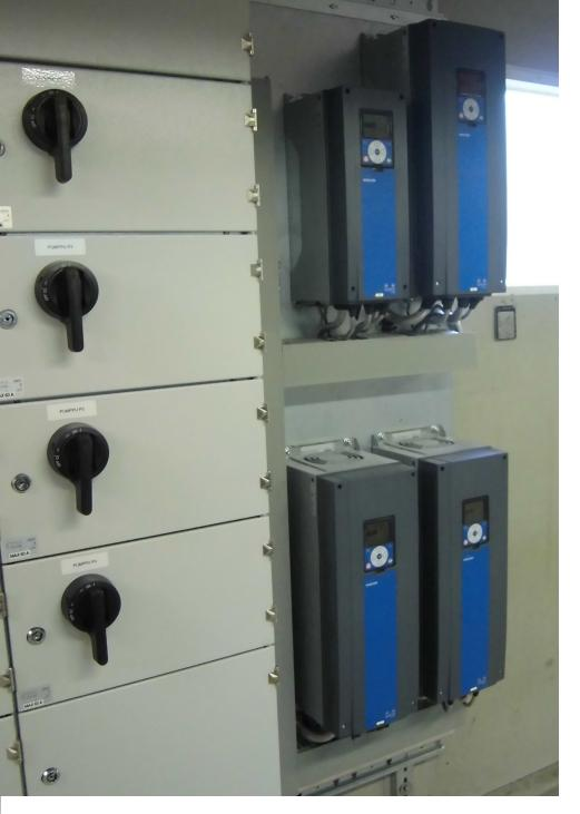
VACON® 100 FLOW units at the Osvald waste water pumping station. The drives were installed on a backplate at SK-kojeisto, the Seinäjoki, Finland based company that has built the switchboards used at KRŚ-Veśi.
