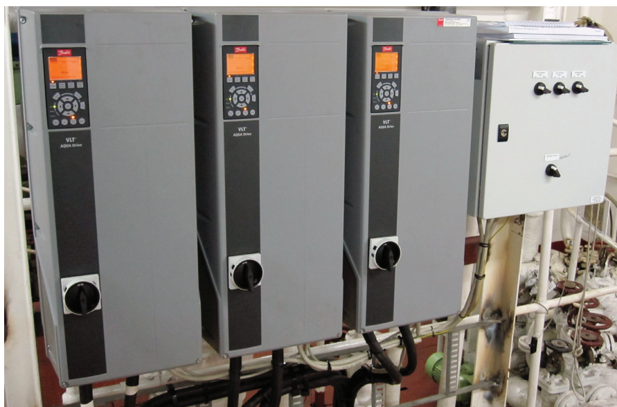
The solution at Dampskibsselskabet NORDEN A/S consists of 3 VLT® AQUA Drive FC 202, 45 kW frequency converters with a cascade pump controller, an electrical switch box for control, and two temperature transmitters.
