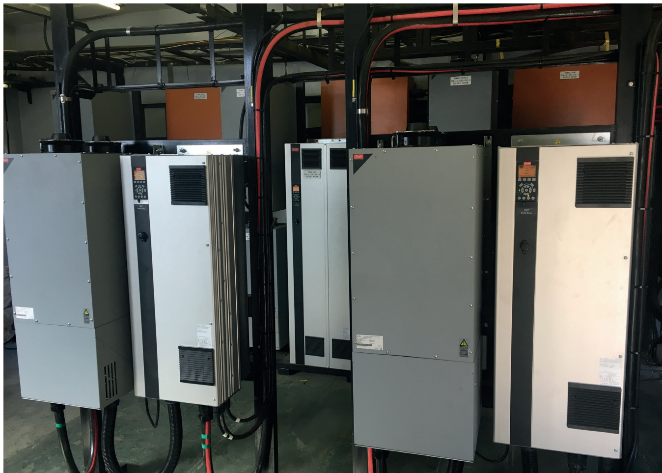
The process cooling water (PCW) system now benefits from VLT® AQUA Drive controlling each of three cooling water pumps, and VLT® HVAC Drive controlling both the cooling tower fans.
