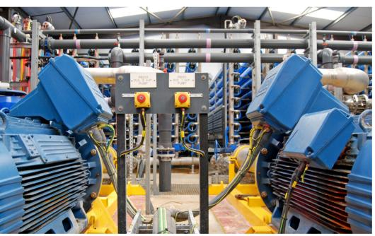
The upgrade involved the installation of a large number of new pumps, almost all of which would need to be controlled by AC drives.
