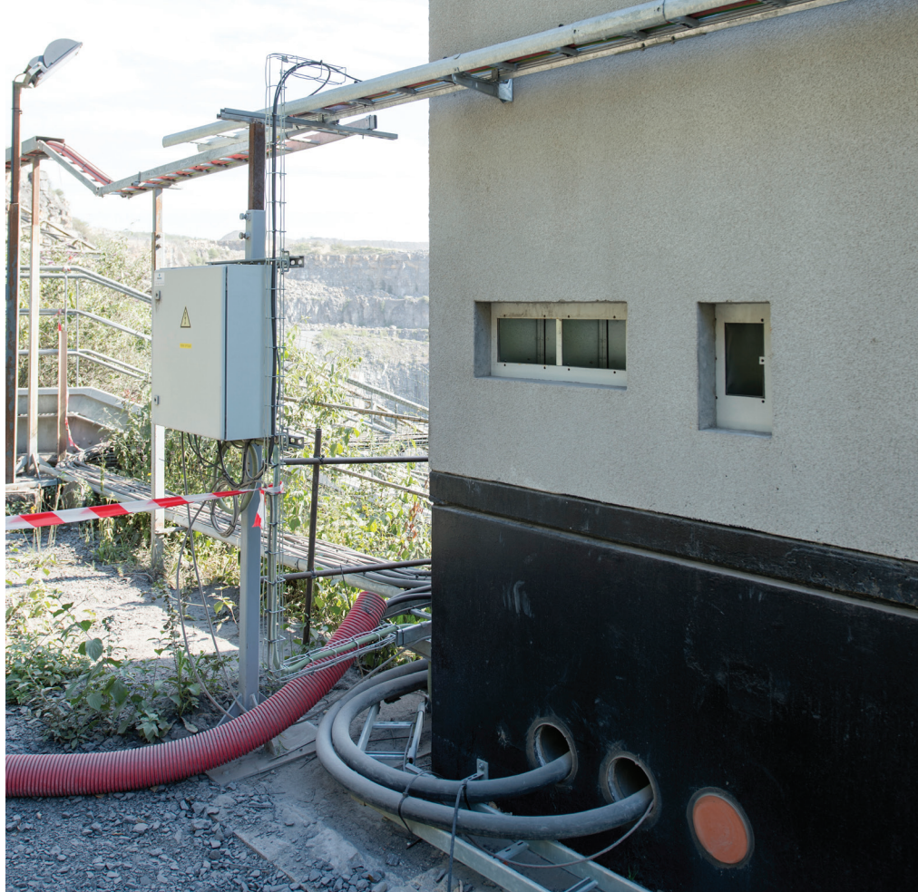
90% of the heat generated by the AC drive bypasses the technical room.
