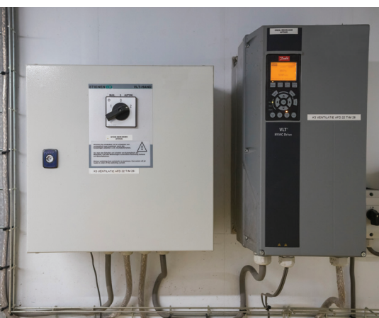
▲ A robust IP55-rated VLT® drive controls the Stienen climate solution equipment.
