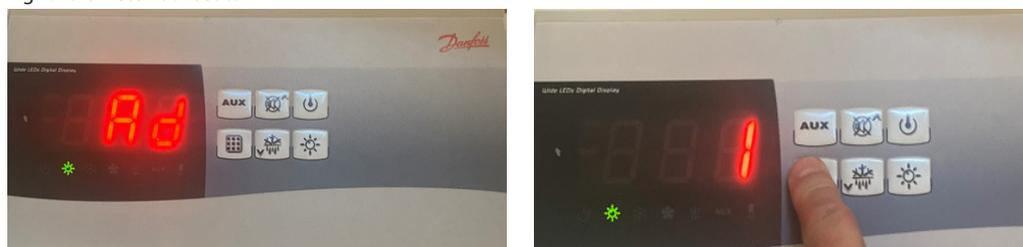
Check that all the default parameter values within the Optyma cold room control are set to site specific requirements – please note that the default alarm delay is factory set to 120 mins the high temperature alarm is set to +99 and the low temperature alarm is set to -99.
