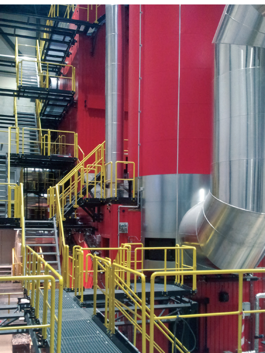
Vertical biofuel boiler and flue gas shotblast cleaning.
