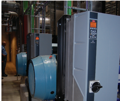
IE4 SynRM motors equipped with VLT® AutomationDrive FC302 frequency converters.
