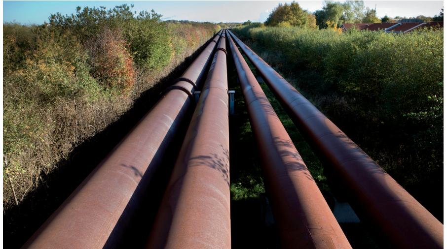
Transmission pipes, district heating in the Aarhus area. source: www.affaldvarme.dk
