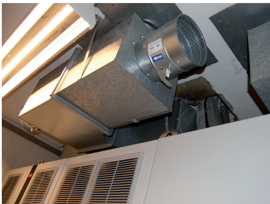
The back channel cooling system of the VLT® AQUA Drives is directly connected to the control room ventilation system.
