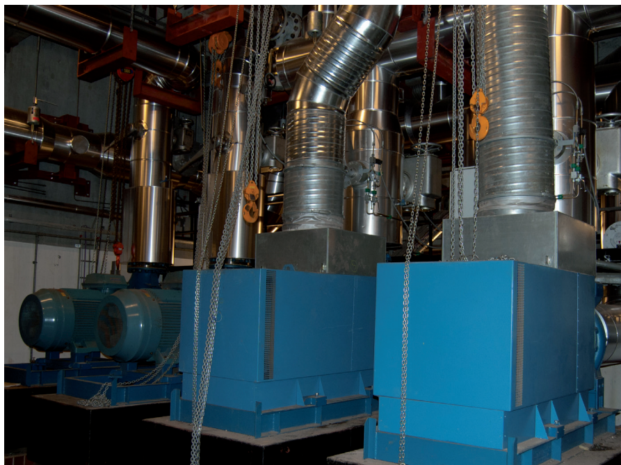
The two 500 kW primary pumps are equipped with two new Danfoss VLT® AQUA Drive FC 202 frequency converters.
