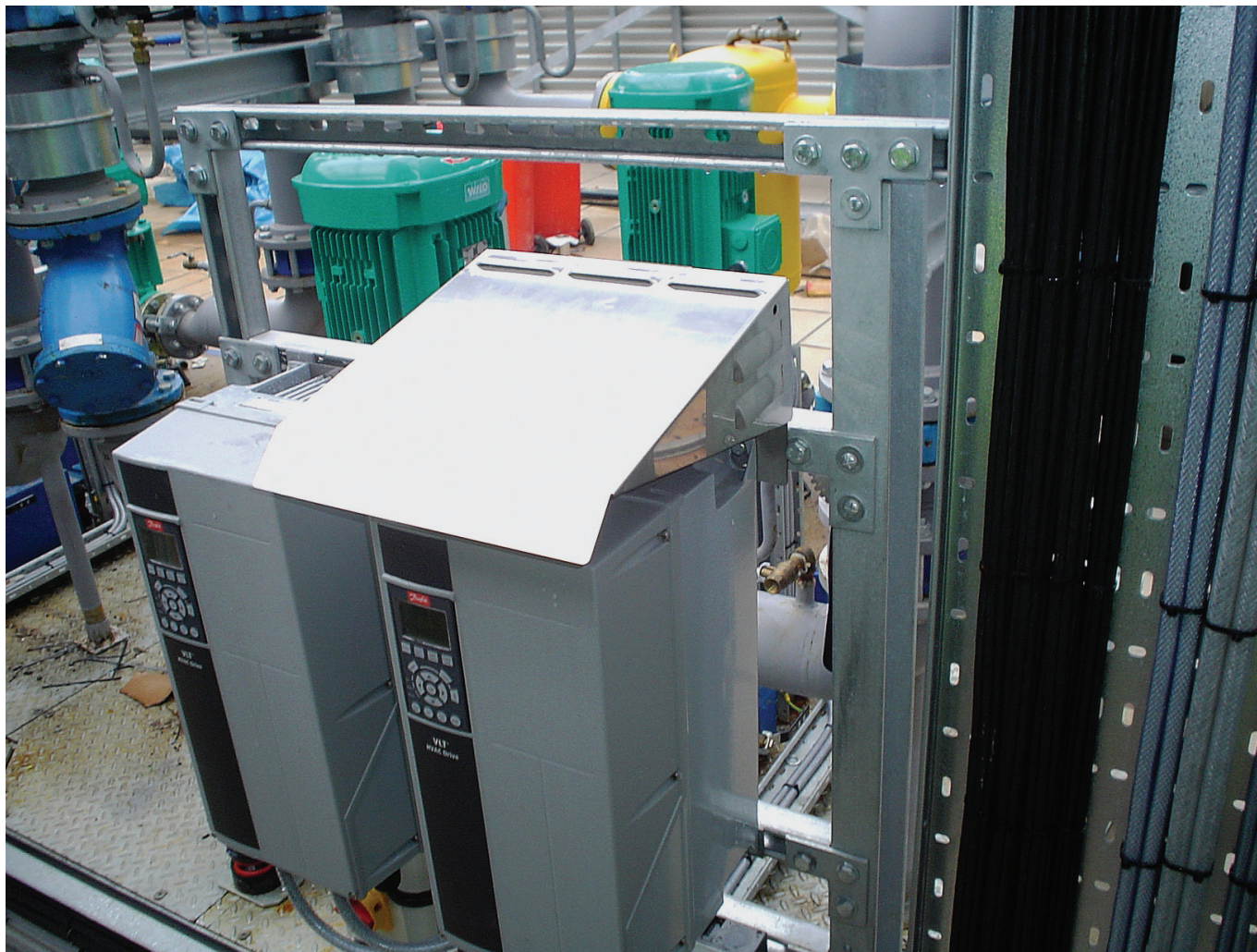
Danfoss FC series can withstand even the harshest pressure washing environments. A NEMA/UL Type 4X rated enclosure provides maximum mounting flexibility
