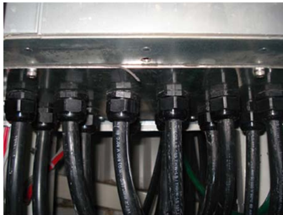
Figure 3.25: Example of proper installation of the gland plate.
