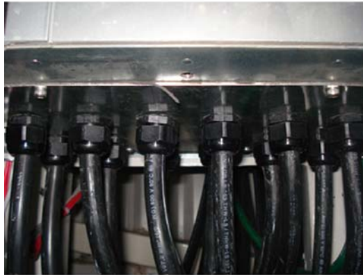
Figure 3.35: Example of proper installation of the connector plate.
