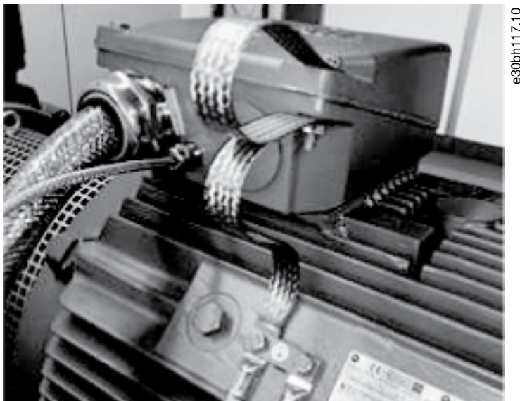
Illustration 17: Installation of EMC straps from the Terminal Box to the Motor Frame
