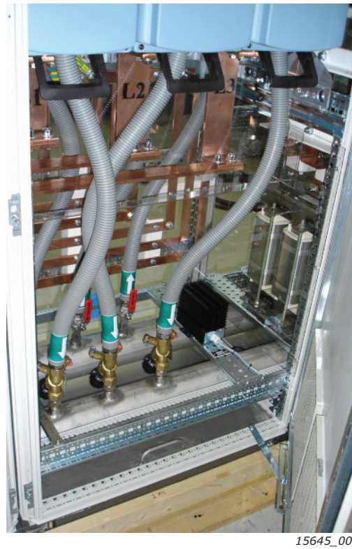
Figure 30. Example installation of water hoses
