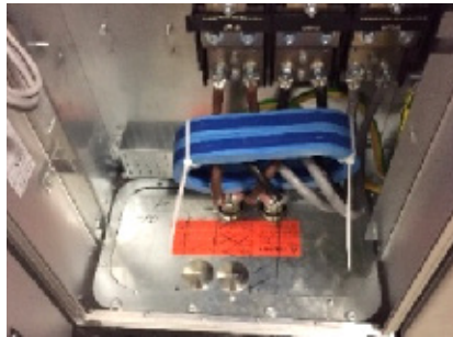
Fig. 6.21 Common-mode cores installed at the drive terminals
