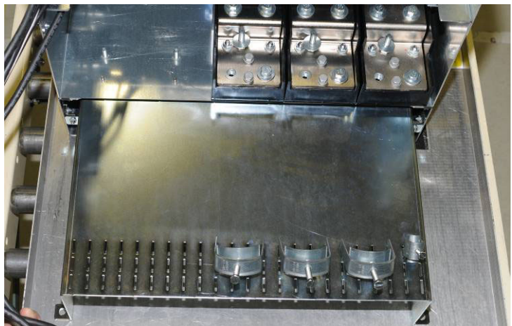
Figure 11. Cable-clamp bracket mounted on E2 frame.
