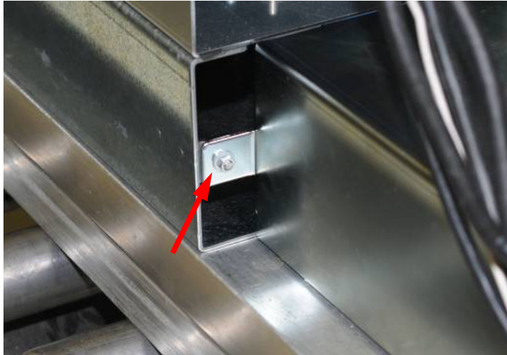
Figure 9. Cable-clamp bracket mounted on mounting tab, left side of E2 frame.
