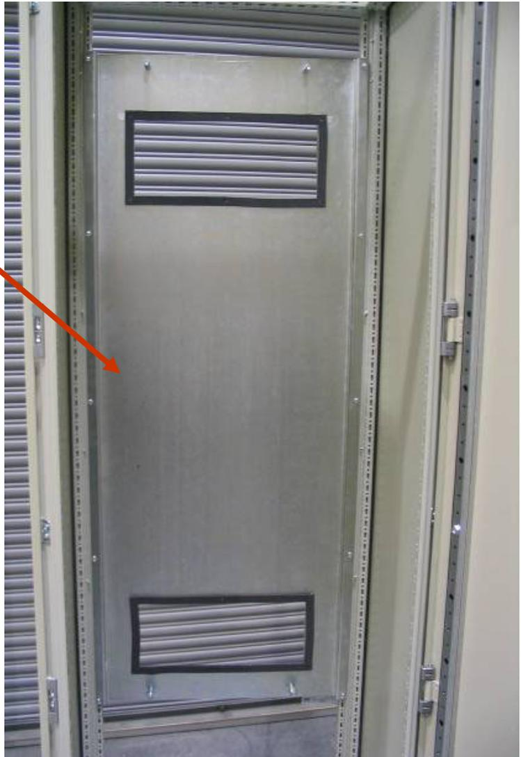
Use the drive mounting plate as a template to mark the openings for the air intake and exhaust along with mounting screw holes on the rear panel of the enclosure.
