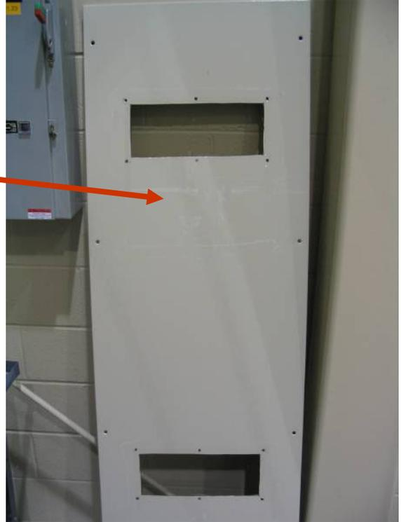
Install gasket material on both sides of the drive mounting plate.
