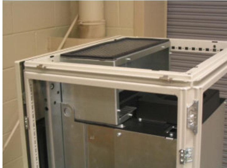
Photo 15. Top duct installed.
