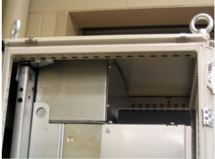
Photo 18. Enclosure top installed.
