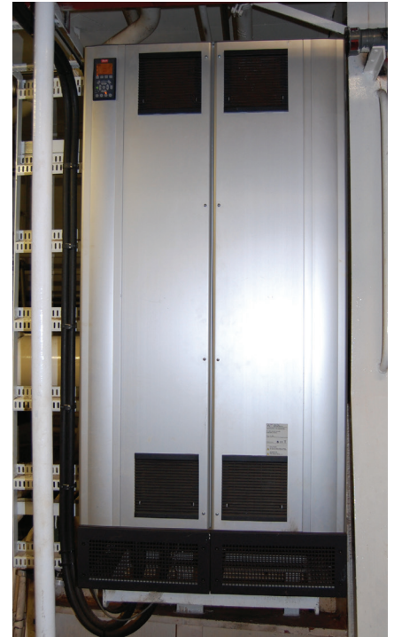
One of the two 190 A VLT® Advanced Active Filters controlling the power system.
