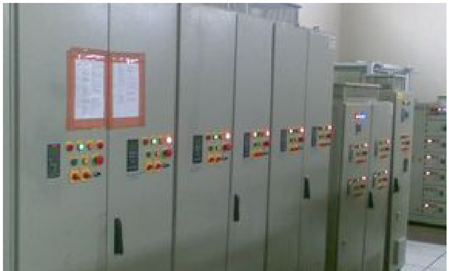
Line-up of VLT® drive panels
