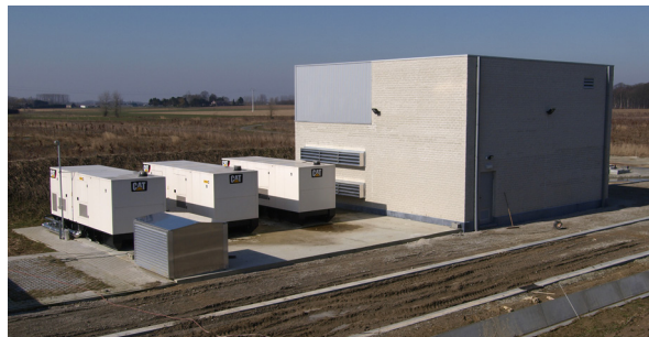
There is a low level of noise generation outside the building because of noise absorbing exhaust ducts.
