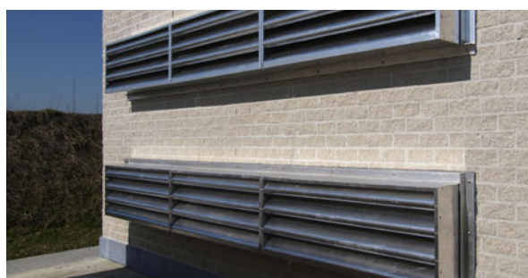
There is a low level of noise generation outside the building because of noise absorbing exhaust ducts.
