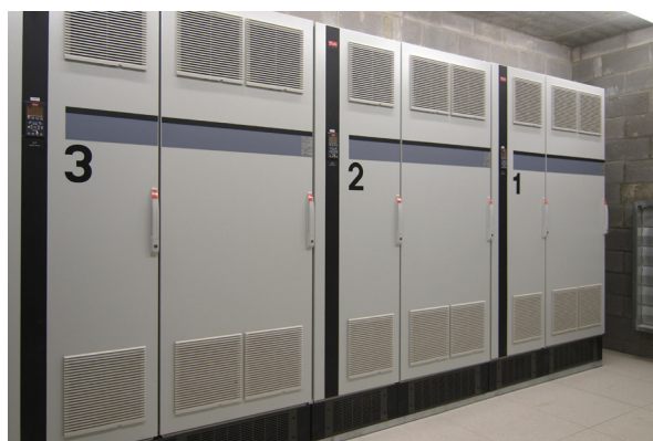
The 3 x 500 kW VLT® AQUA Drives standing side by side. The room is just wide enough to contain all three.
