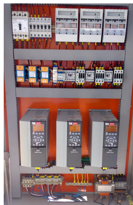
The VLT® AQUA Drive controls motor speed in accordance with pumping requirements.
