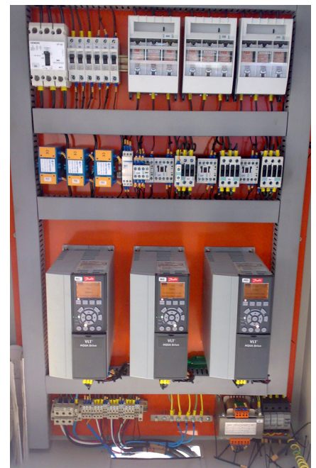
The VLT® AQUA Drive controls motor speed in accordance with pumping requirements.
