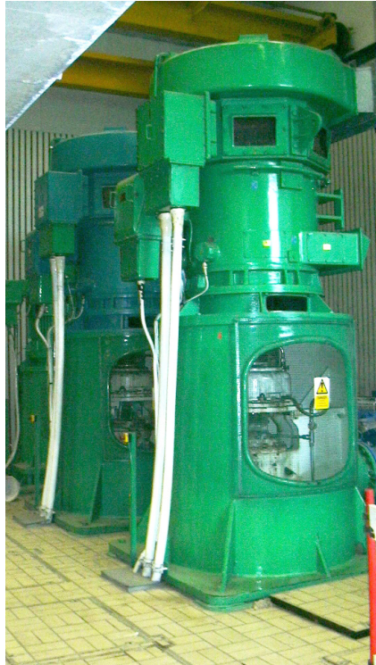
3 remaining 3.3 kV pumps under consideration for frequency converter control
