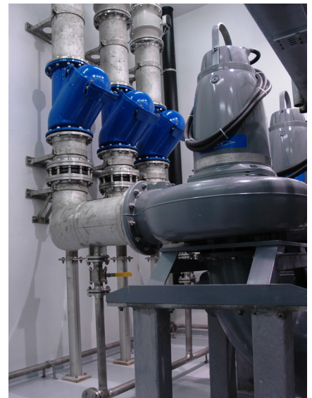
Three Flygt pumps controlled by a PLC raise wastewater from a reservoir for it to flow by gravity alone to the next pumping station.
