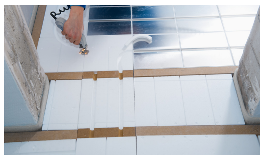
Fig. 6: Where required cut individual pipe channels using the SpeedUp hot wire cutter.
