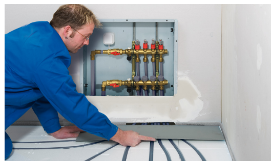
Fig. 10: Cover pipe work in front of manifold with SpeedUp load bearing steel to protect against damage.
