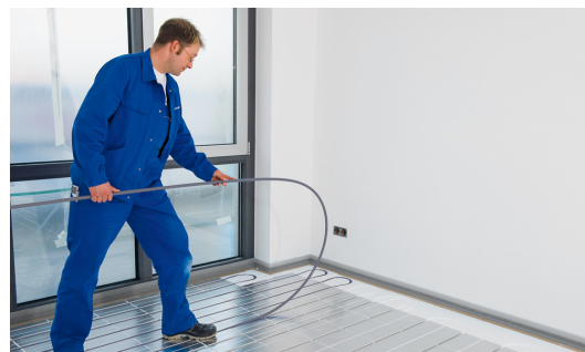
Fig. 8: Holding the pipe in a large curve to avoid tension, press the composite pipe into the channels. Avoid lifting pipe once installed in the header panels.
