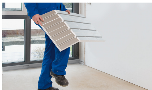
Fig. 4: Snap the pre-scored heat panels as required.
