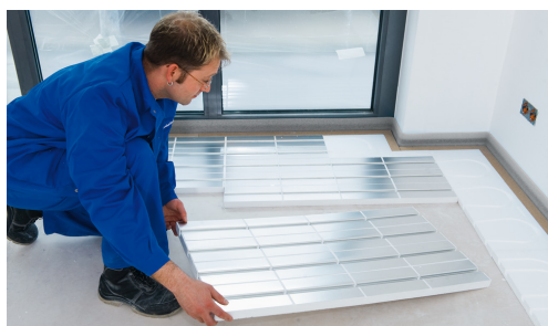
Fig. 3: Place the SpeedUp heat panels (CZ: pipe distance 250 mm, EZ: pipe distance 125 mm). Fill gaps and unheated areas with blank panels.
