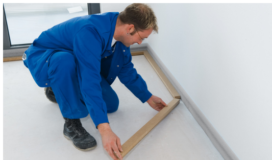
Fig. 1: Install SpeedUp perimeter insulation and support batten on dry, even and load bearing substrate.
