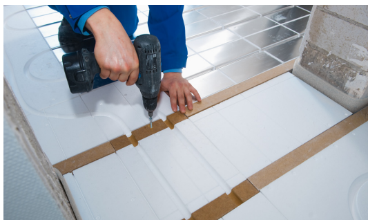
Fig. 7: Support battens in thresholds should be screwed down.
