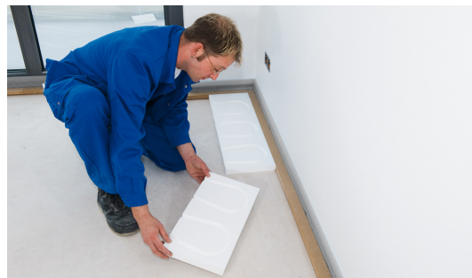
Fig. 2: Following the layout, begin the installation in one corner with a SpeedUp header panel.
