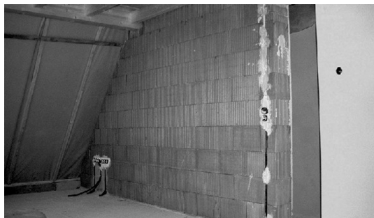
Fig. 1: Inspection of the pipe wall. Remove unevenness and create a flat surface.
