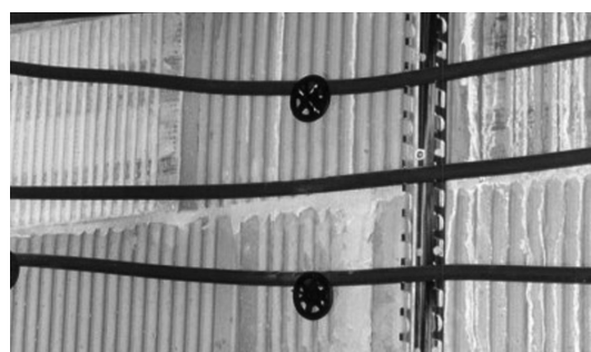
Fig. 6: Drill at least 8 holes for wall dowels (70 mm) per m 2 and attach bottom section of dowel.
