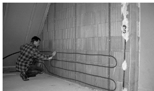
Fig. 4: In accordance with the laying procedure push composite pipe into the rails from bottom to top, starting with the supply line below.
