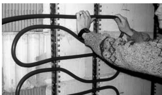
Fig. 5: In doing so do not exceed the maximum pipe bend length of 20 cm.
