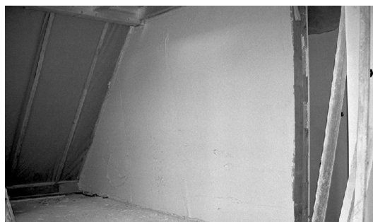
Fig. 10: The applied layer of plaster can be smoothed or matted as required.
