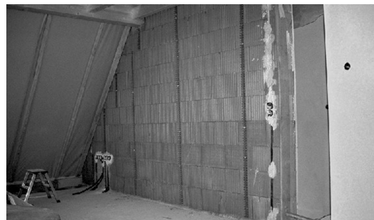
Fig. 2: Start by laying the rails vertically with a spacing of maximum 1 m.
