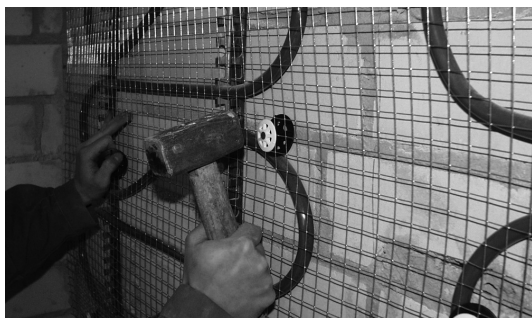
Fig. 7: Attach wall heating metalgrid from top to bottom, lightly tensioned with 10 cm overlap, using the dowel upper section.
