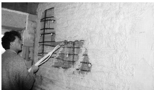
Fig. 9: Spray on the plaster in a single 35 mm layer from the top to bottom according to the manufacturer's instructions.
