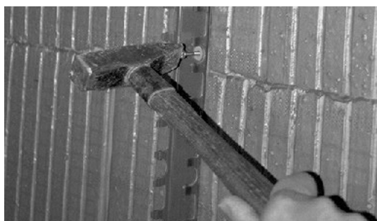
Fig. 3: Attach the rails in three places with hollow wall anchor-/nailed dowels and screws.
