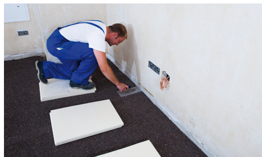
Fig. 8: Compound at the edges may have to be worked again with trowel.
