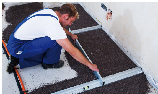
Fig. 7: In larger rooms the leveling of the compound will have to be finished in several adjacent lines.
