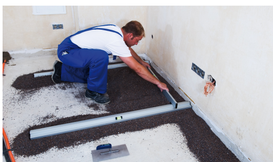
Fig. 5: Continue to fill the floor in sections with compound and then position the leveling rule on the parallel guides.
