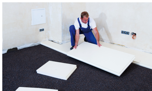
Fig. 10: Once finished begin laying of the additional insulation.
