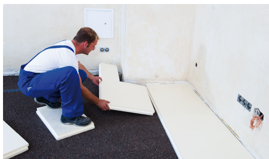
Fig. 9: Insulation panels serve as walk boards or walk islands and so prevent damage.
