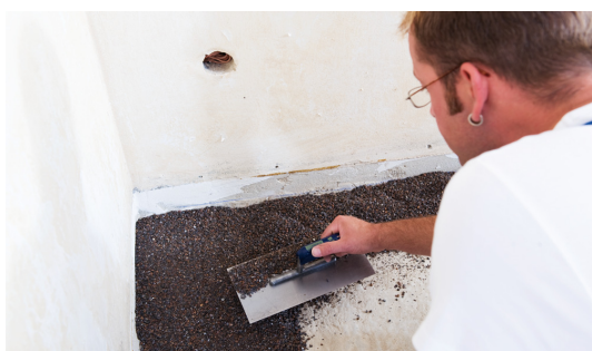
Fig. 3: With large flat trowel spread and flatten the compound.
