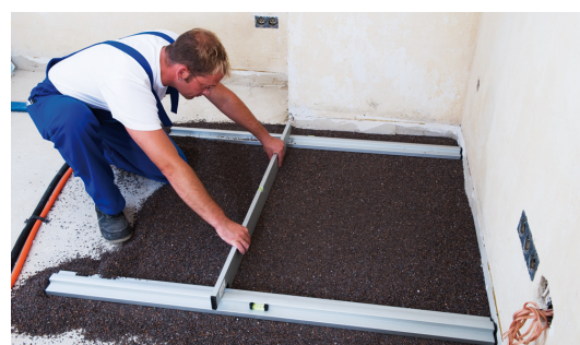
Fig. 6: During the leveling additional compound may be required.
