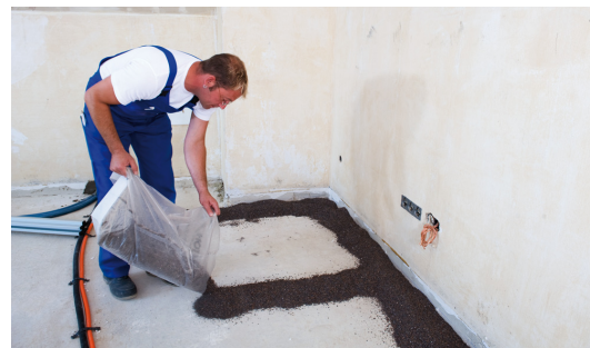
Fig. 2: Pour lines of compound to a moderate height, the distance of the lines depending on the width of the leveling rule.
