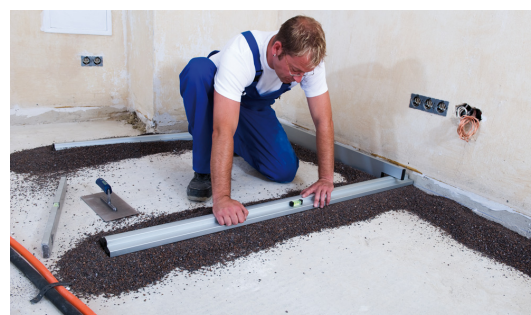
Fig. 4: Position the parallel guides on each of the lines and adjust according to the required height.
