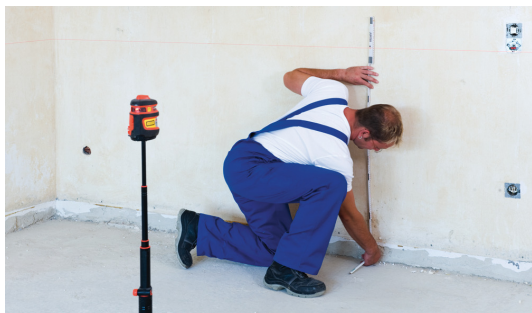
Fig. 1: Determine your datum and your compound level (min. 10 mm, max. 60 mm).
