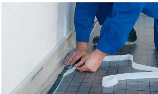
Fig. 5: Attach connection tape of Basic perimeter insulation avoiding tension and tears in the corners.
