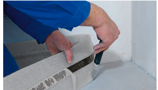
Fig. 2: Score lightly Basic perimeter insulation 3 cm from below, at inside corners on wall side, at outside corners on room side.
