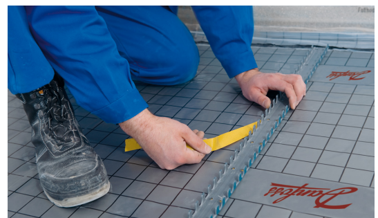
Fig. 6: Position BasicRails according to lay-out. Use pipe cutter to shorten the rail to required length.
