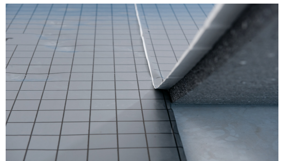
Fig. 4: Care should be taken when laying the overlapping panels. Tape butt joints and tape lap joints when using liquid screed.
