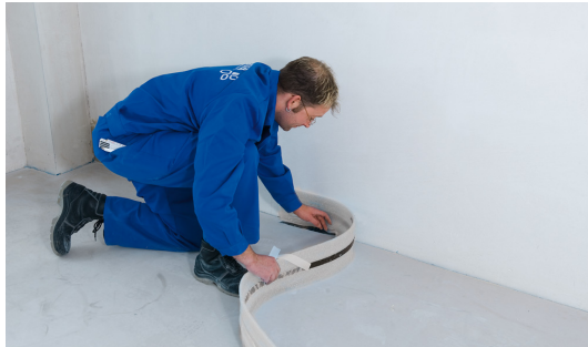
Fig. 1: Attach the selfadhesive Basic perimeter insulation tape on the wall. 1
