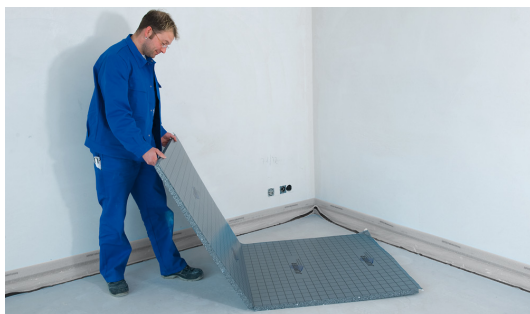
Fig. 3: Begin laying Basic insulation overlap panels with the flap against the wall.
