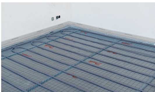
Fig. 9: Only use connectors on straight sections of pipe and not bends.
