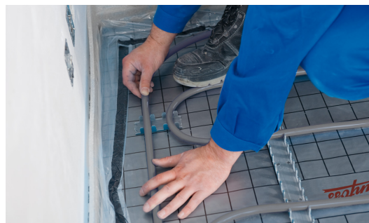
Fig. 8: Fix flow and returns every 2 m with clips. Maximum distance from pipe bend and clip is 25 cm.
