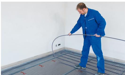
Fig. 7: Install pipe in wide curve and tension free as illustrated and according to lay-out.
