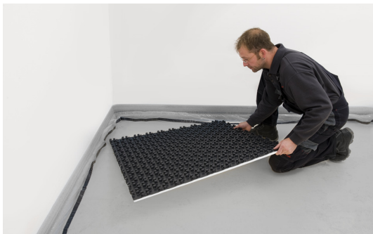
Fig. 3: Lay this BasicGrip panel in the left hand corner of the room.
