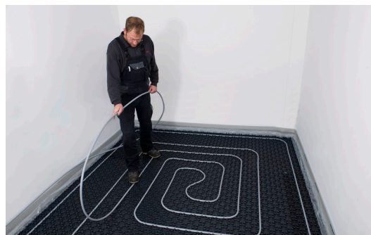
Fig. 8: Lay pipes in snail form, at first with double spacing in order to maintain the calculated pipe distances.
