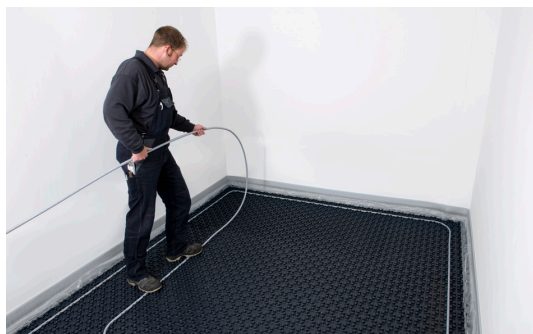
Fig. 7: The pipes can be laid by one person by using the pipe dispensing wheel.
