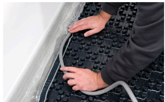
Fig. 6: When using liquid screed, seal off the foil strips of the perimeter insulation with PE-string. On cement screed, the foil is loosely placed on the studded panel.
