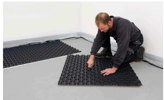
Fig. 4: Install the studded panels one over the other. Cut wall side overlapping edges off. Cut the last panel to fit.
