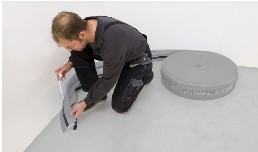
Fig. 1: Attach the perimeter insulation with tape on wall. 1
