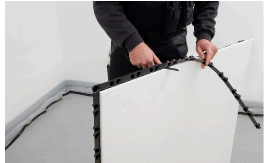
Fig. 2: Cut off overlaps on both ends of the first BasicGrip panel.
